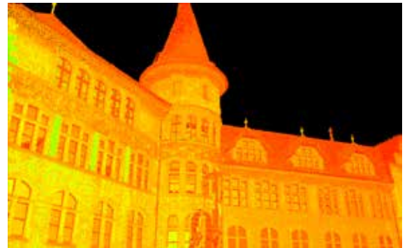
Figure 2: Laser scan of a building provides a lot of detail. Literally this view shows in context millions of measurements; together, they look like a photograph.
